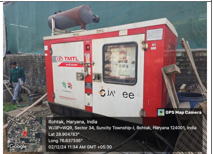
Fig: 15 kVA Genset installed at site
